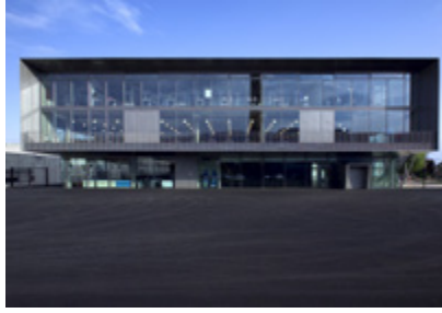
CENTRAL BUILDING, ORBE, 2006
